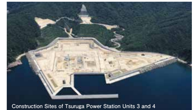
Construction Sites of Tsuruga Power Station Units 3 and 4
